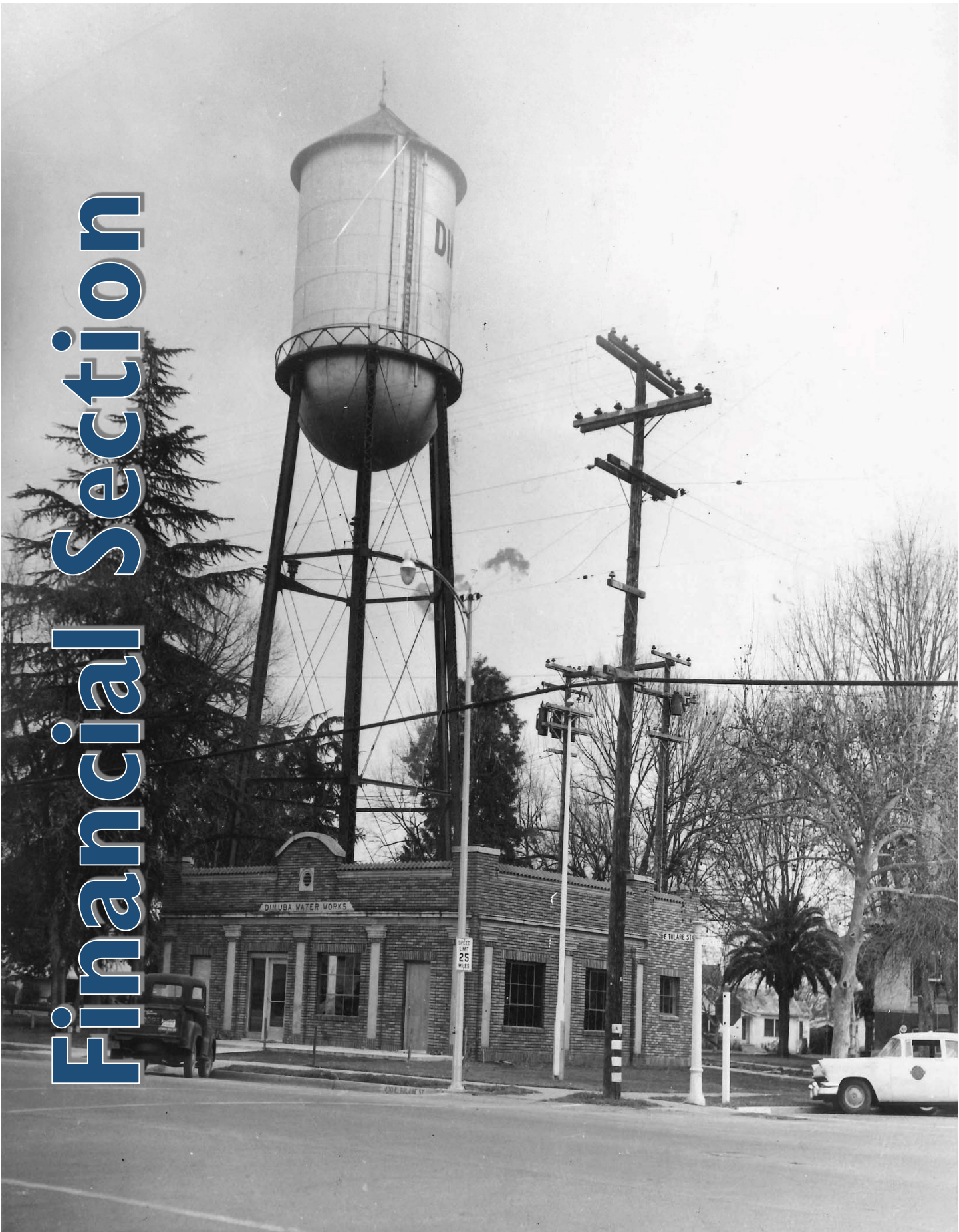
Dinuba Old Water Tower
